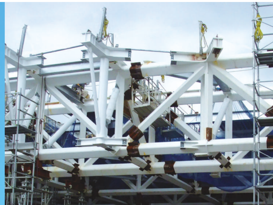
Steel Structure Roof (Square Hollow Section)
